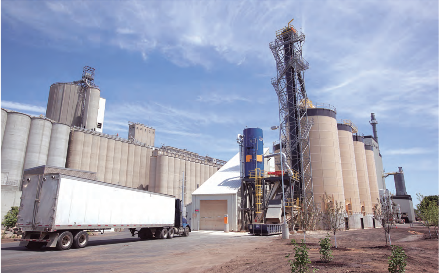
The biomass-fired Koda Energy LLC power plant in Shakopee (above) generates 22 megawatts of power. (Staff photo: Bill Klotz)
